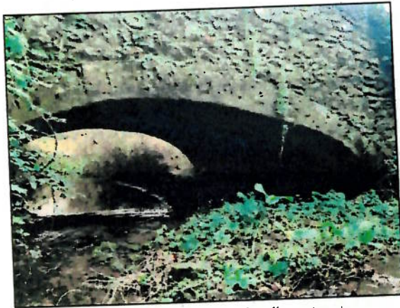
Plate 23 WC4 Stone Arch Bridge - Small crevices in stonework but otherwise solid construction. No evidence of bats. Low roost potential
