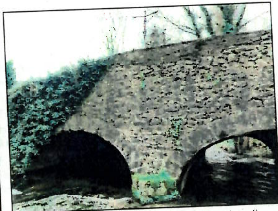
Plate 24 WC5 Stone Arch Bridge - Ivy cover and small gaps present, but underside is smooth concrete. No evidence of bats. Low roost potential
